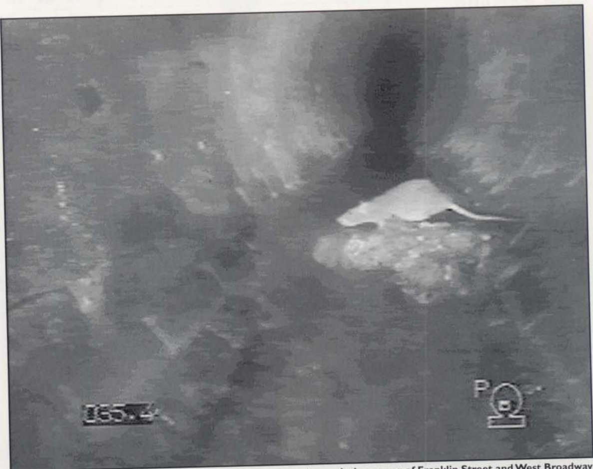
Video image from a robot probe sent to explore the sewers beneath the corner of Franklin Street and West Broadway in New York City.
