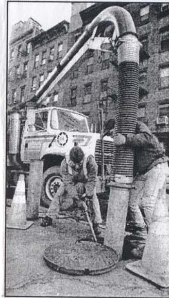
(Above) In mobile studio, Brian Wiprud, left, and Bob Stark observe video transmitted by sewer camera beneath Greenwich Street. (Right) At Hubert and Greenwich Streets, Stark sprays basin, wetting debris sucked up by giant vacuum held by Doug Hamblin. After cleaning, the basin was photographed.
